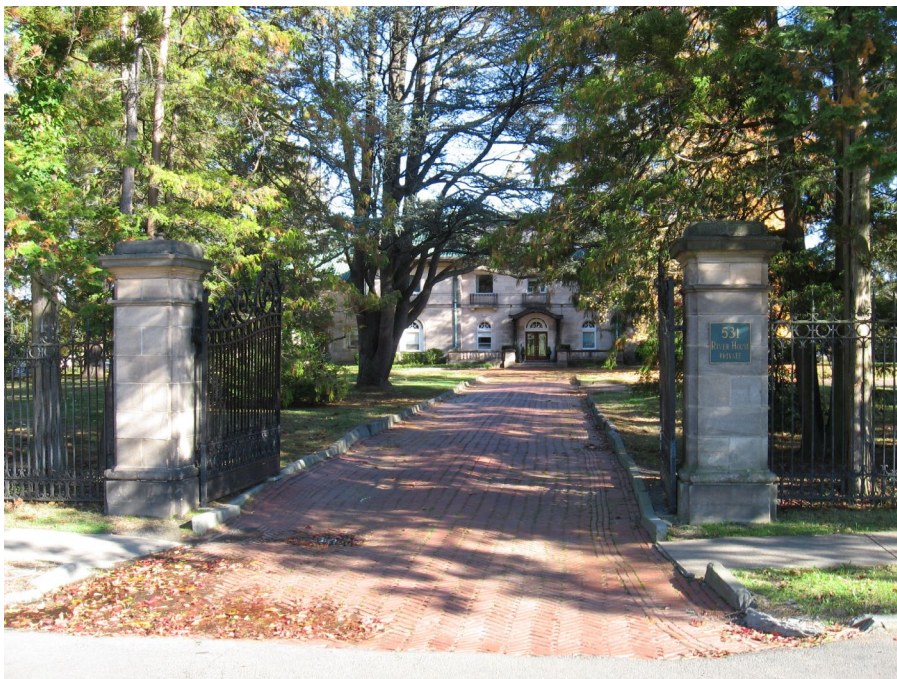
View of 'River House' at 531 North Broadway
