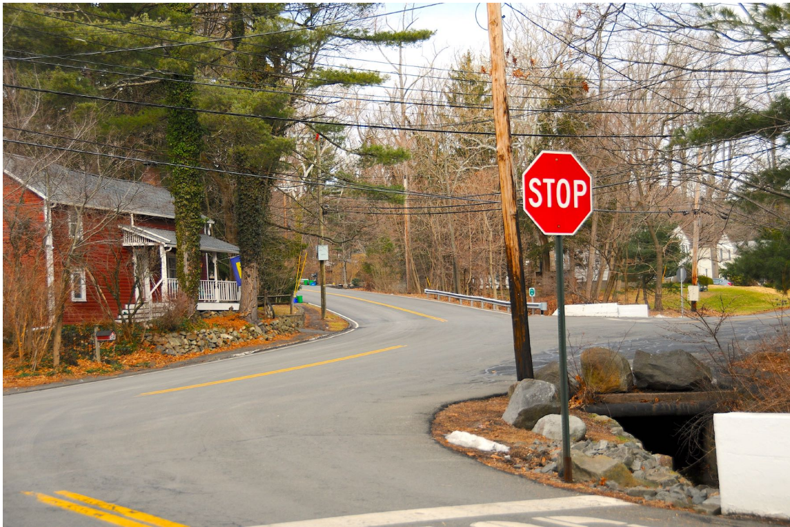
View at Intersection of Midland Avenue and Old Mountain Road
