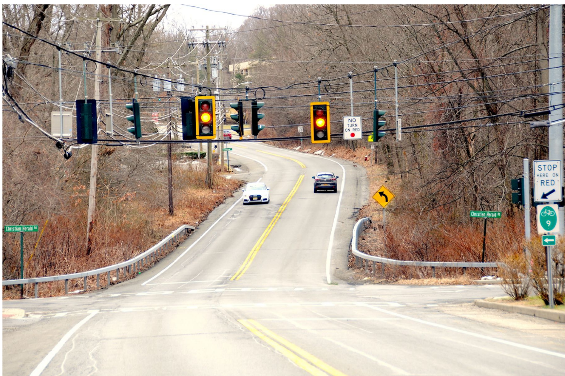
View at Intersection of Route 9W and Christian Herald Road
