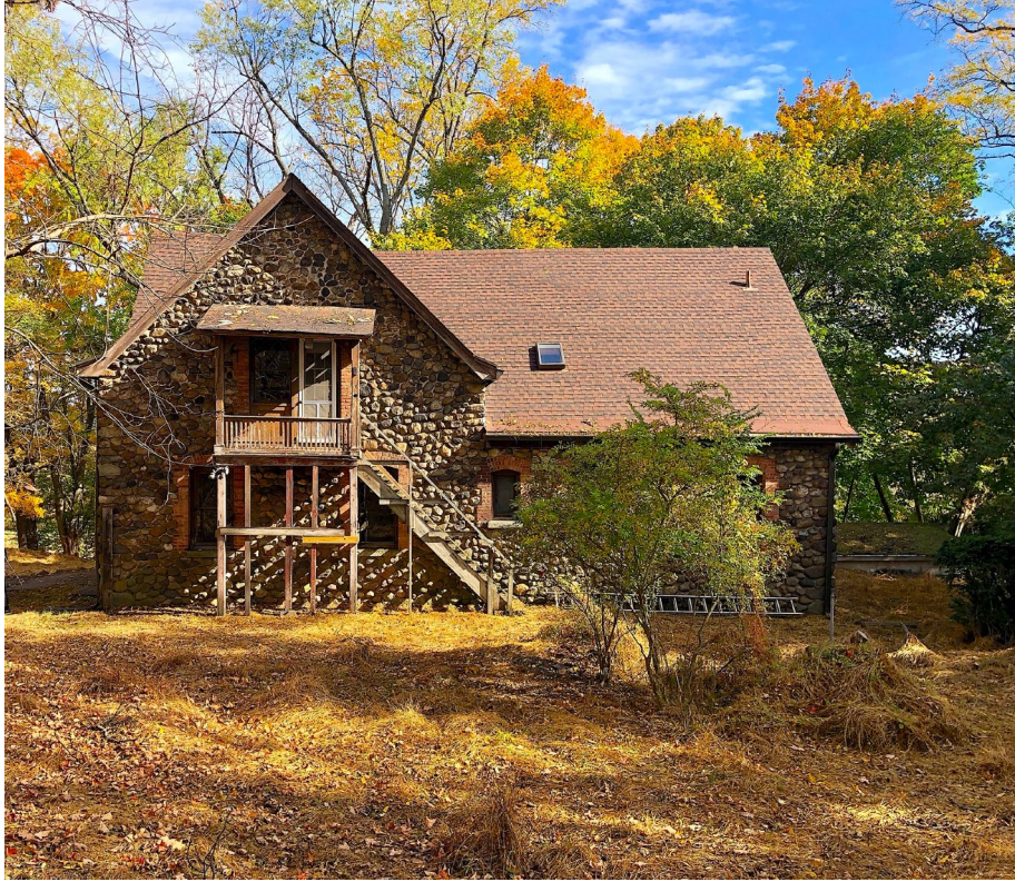
View of Existing Stone House at River Hook
