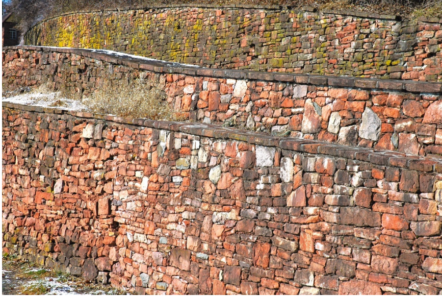
Retaining Walls at Nyack Beach State Park
