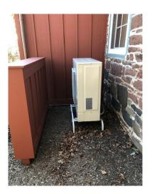
**Clean heating**: In winter, an air source heat pump is a low carbon alternative method to gas. Air source heat pumps extracts ambient heat from outside, heating the refrigerant inside the heat pump. The air is then boosted to a higher temperature using a compressor and then distributed into the interior space.
