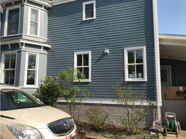
North side of driveway (left side looking in - House side).
