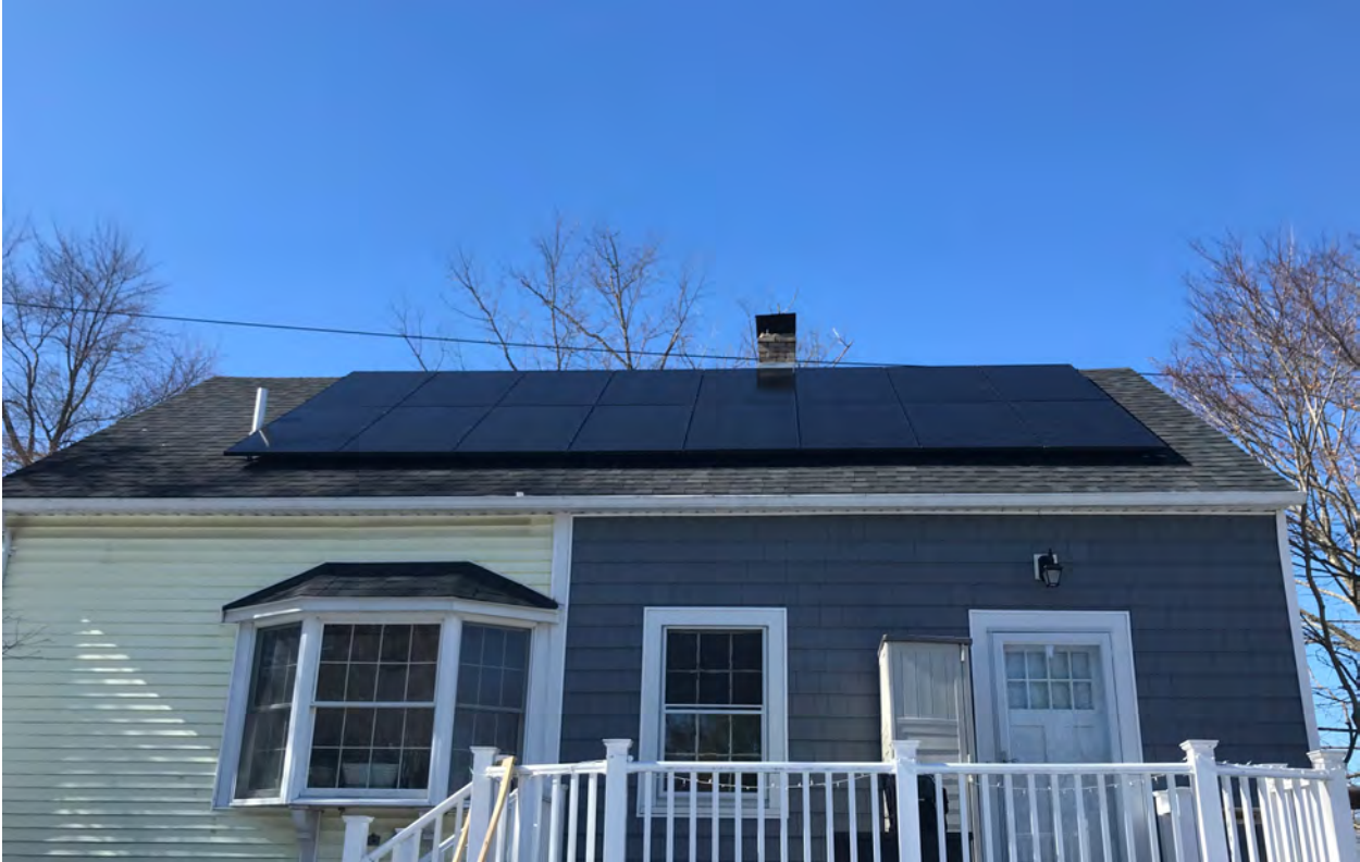
Yassky-Glynn: 214 Radcliff Dr. Nyack, NY 10960 Example of LG-340 panels installed on a roof
