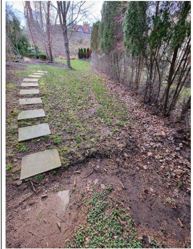
Drainage issue, northern side
