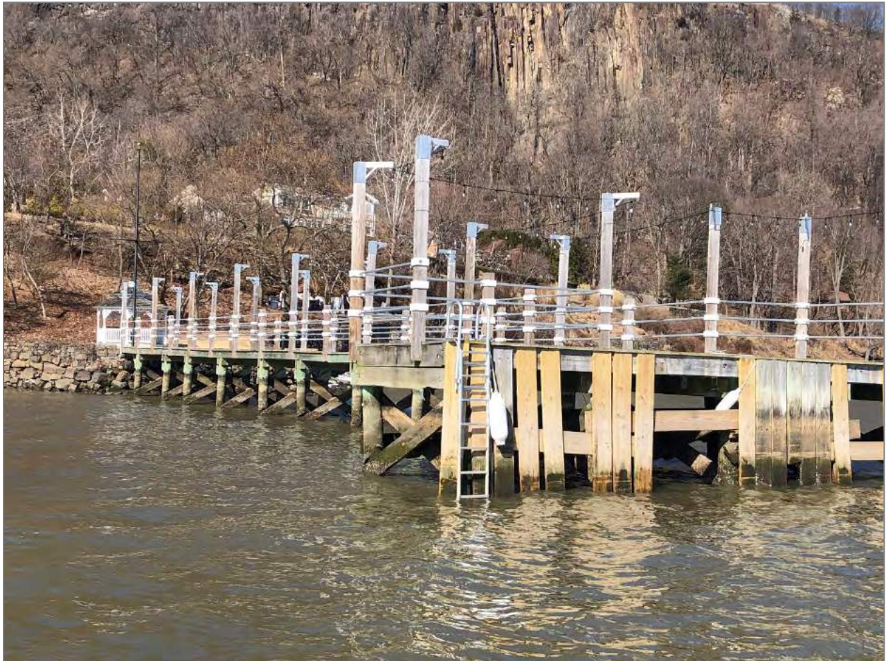
Photograph 9: Existing pier – Facing northwest.
