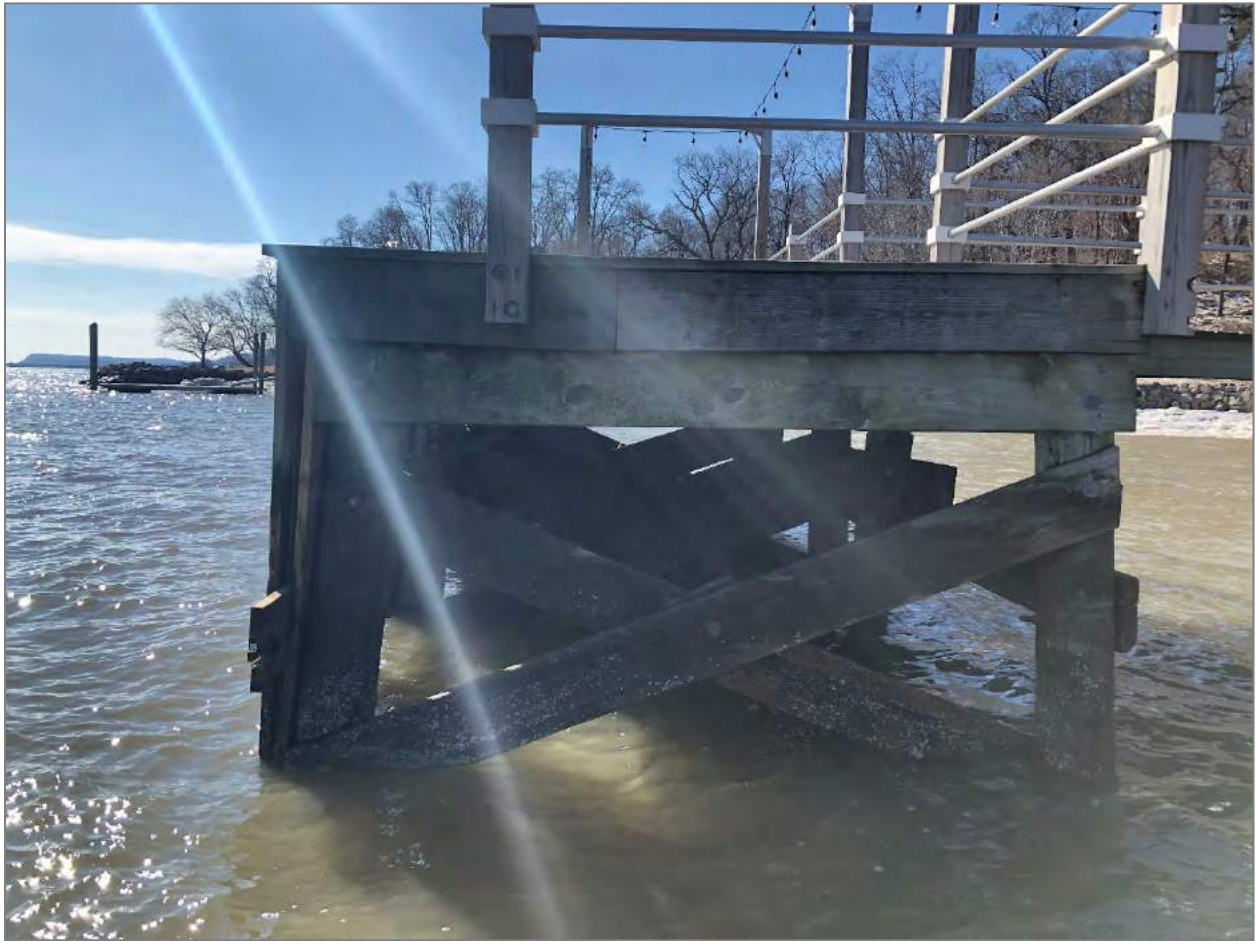
Photograph 10: Existing pier – Facing south.
