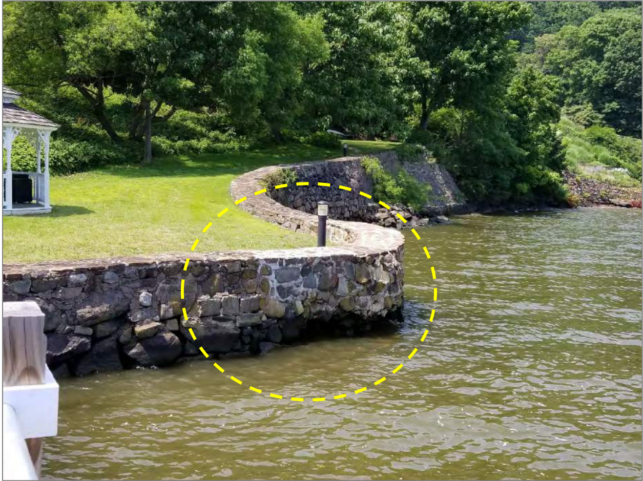
Photograph 3: Existing seawall – Facing northwest.
