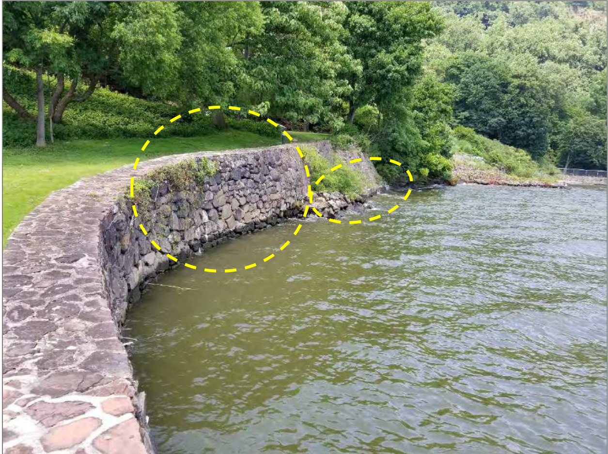
Photograph 1: Existing seawall - Facing northwest.
