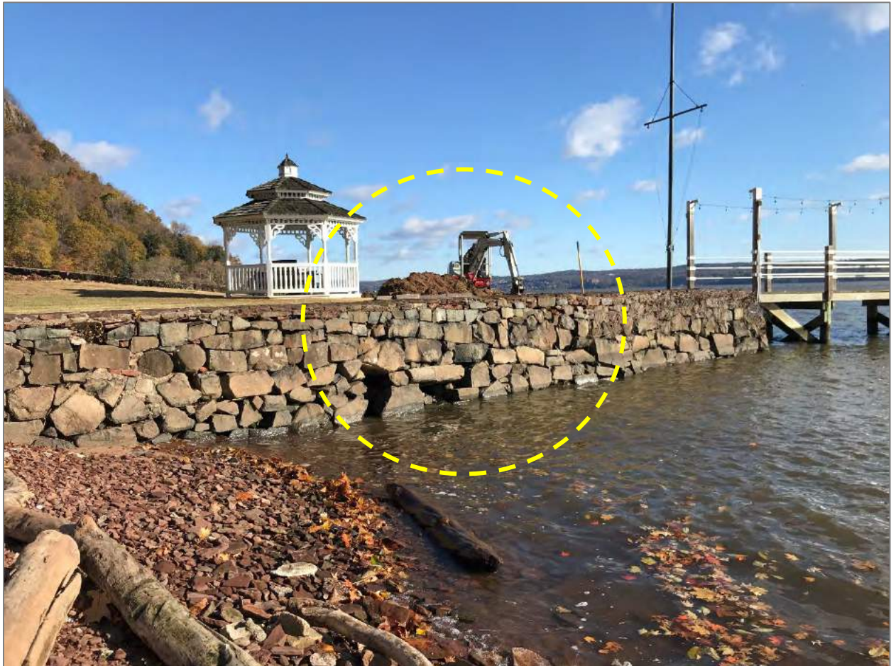
Photograph 13: Existing seawall - Facing north.
