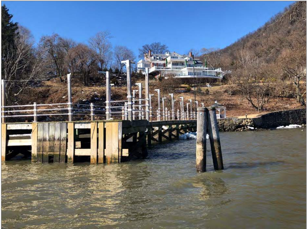
Photograph 8: Existing pier and dolphin – Facing west.
