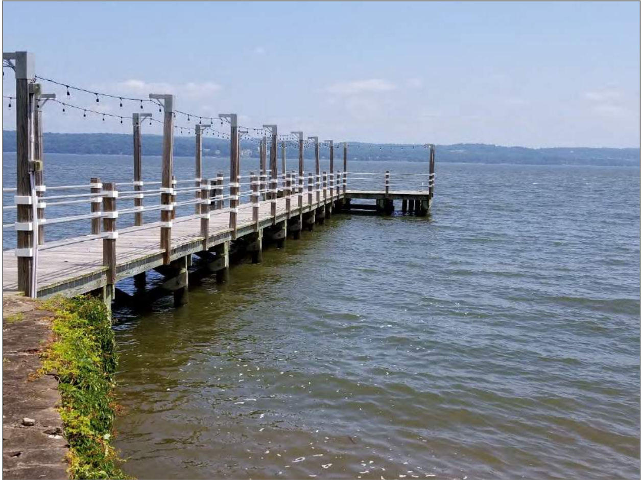
Photograph 7: Existing pier - Facing east.
