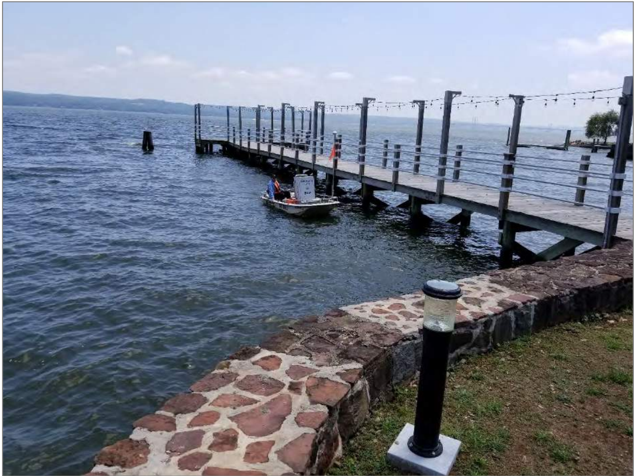
Photograph 6: Existing pier and seawall – Facing southeast.
