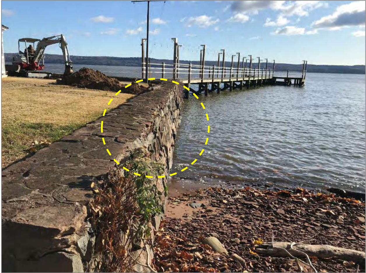
Photograph 14: Existing seawall - Facing east.
