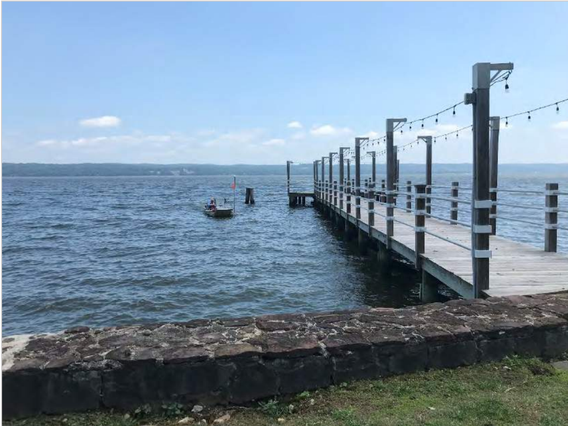
Photograph 1: Existing Pier and Seawall – Facing southeast.
