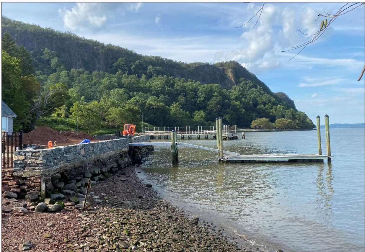
Photograph 1: Existing seawall, pier, and floating dock at low tide, facing north.
