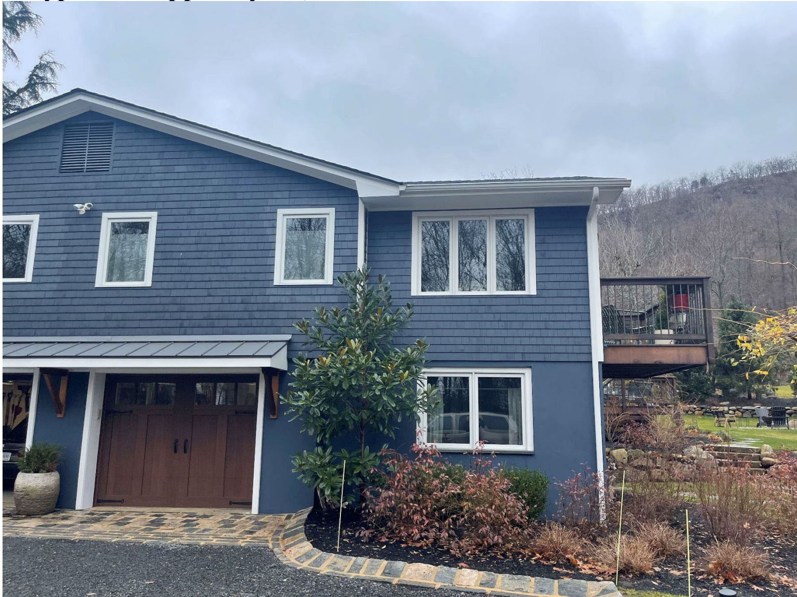
EAST SIDE OF HOUSE
