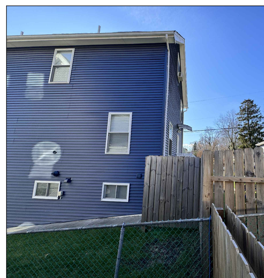
1d EXISTING NORTH FACADE
