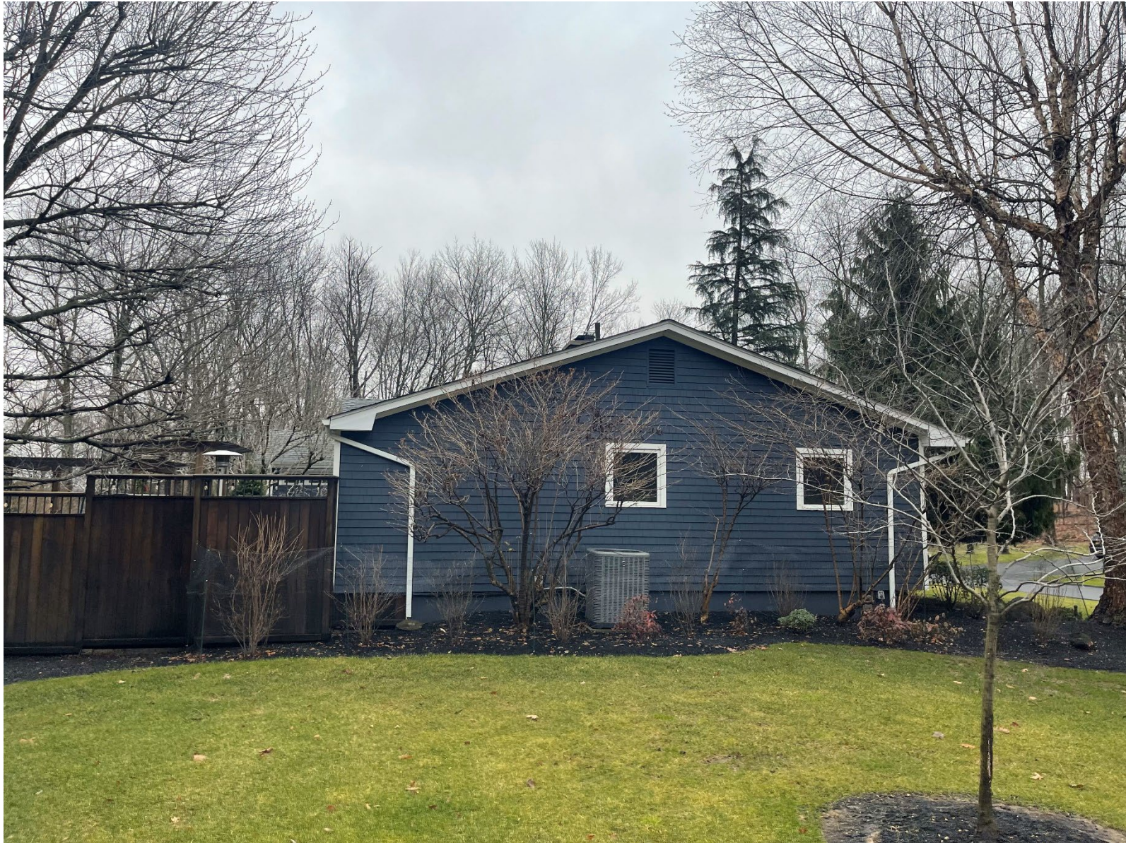
WEST SIDE OF HOUSE
