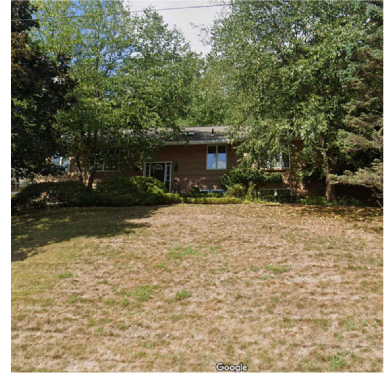
ADJACENT PROPERTY ON THE RIGHT
