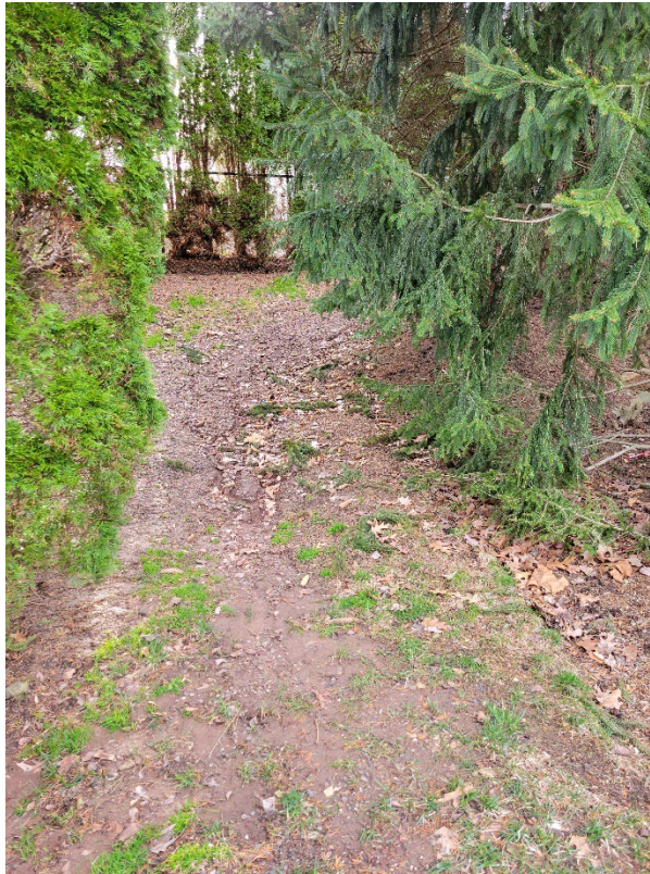
Drainage issue, southern side
