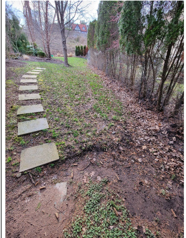
Drainage issue, northern side
