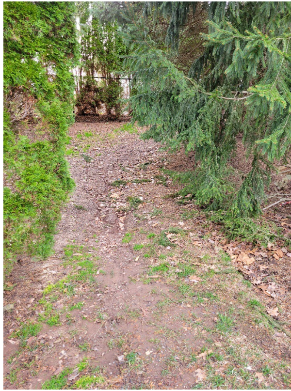
Drainage issue, southern side
