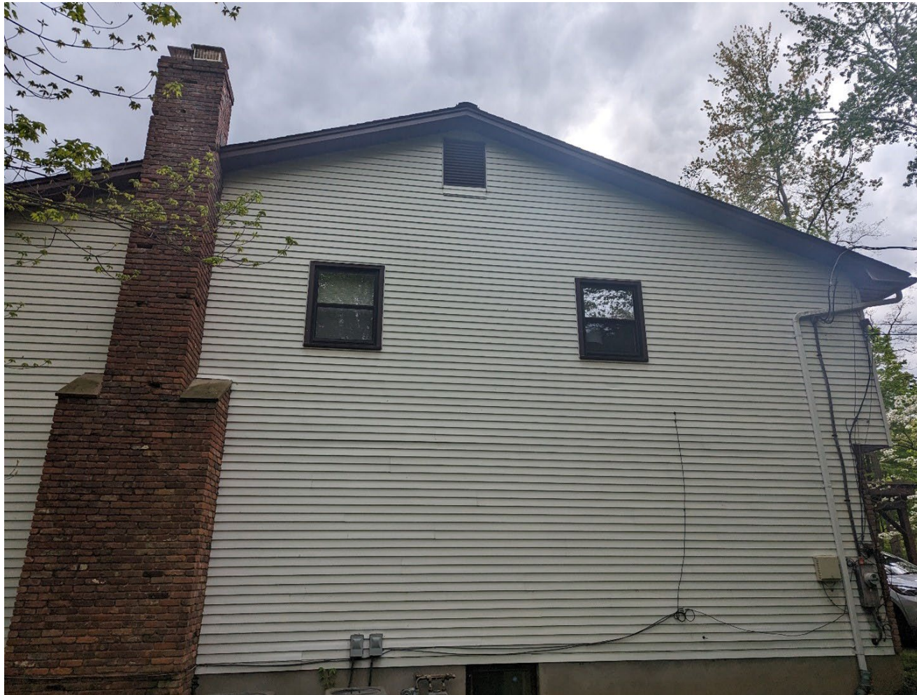
Northern Side of House
