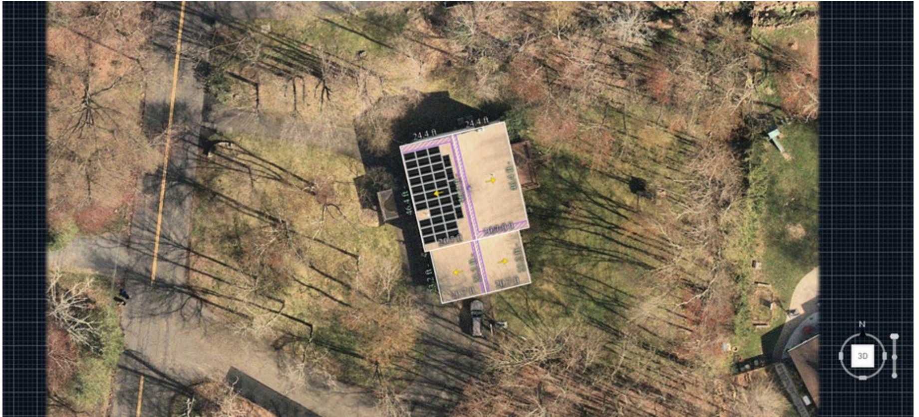
Aerial View of Panels
