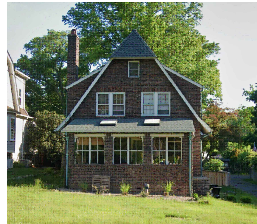
ADJACENT PROPERTY ON THE RIGHT
