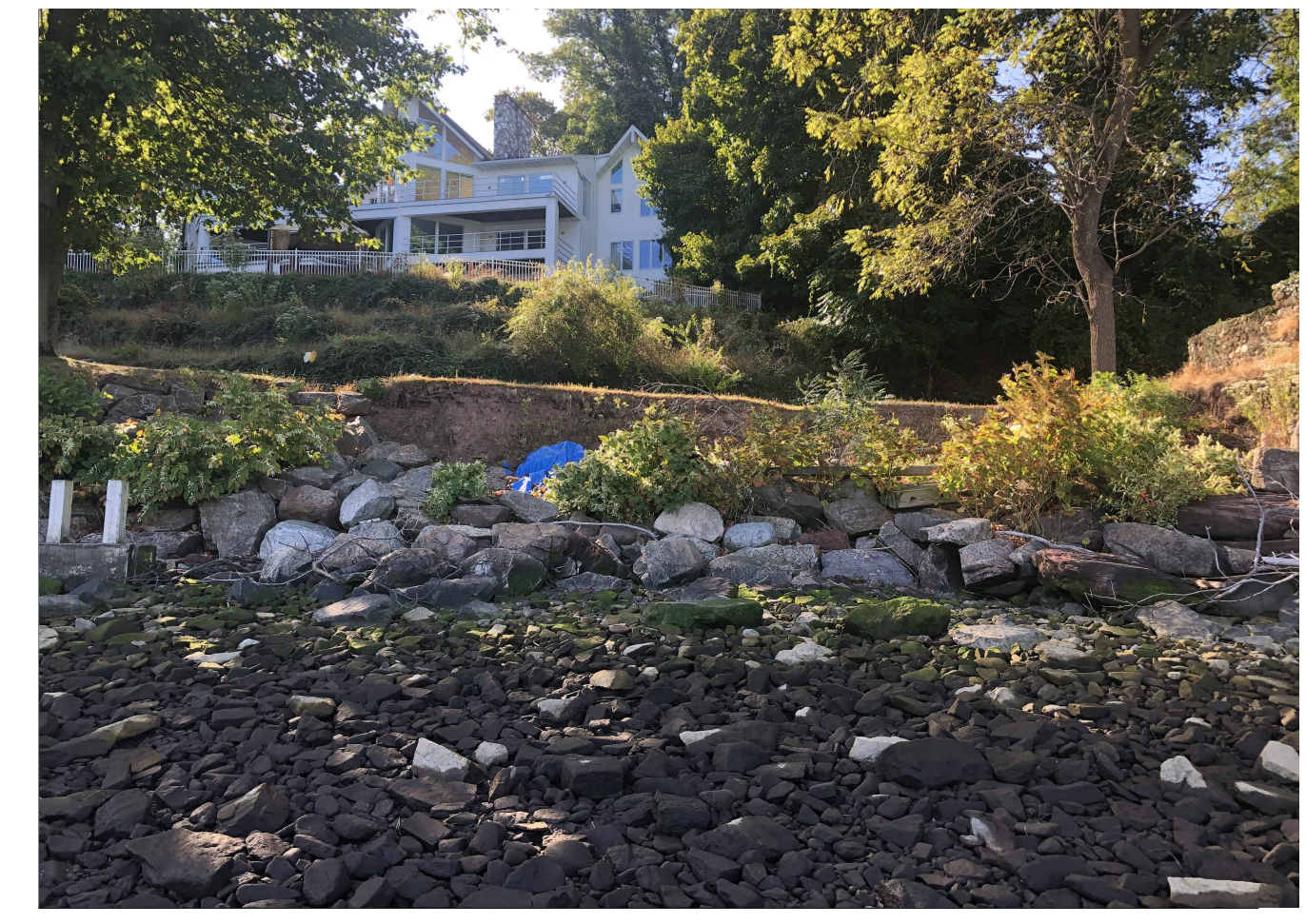
EXISTING SITE CONDITIONS
